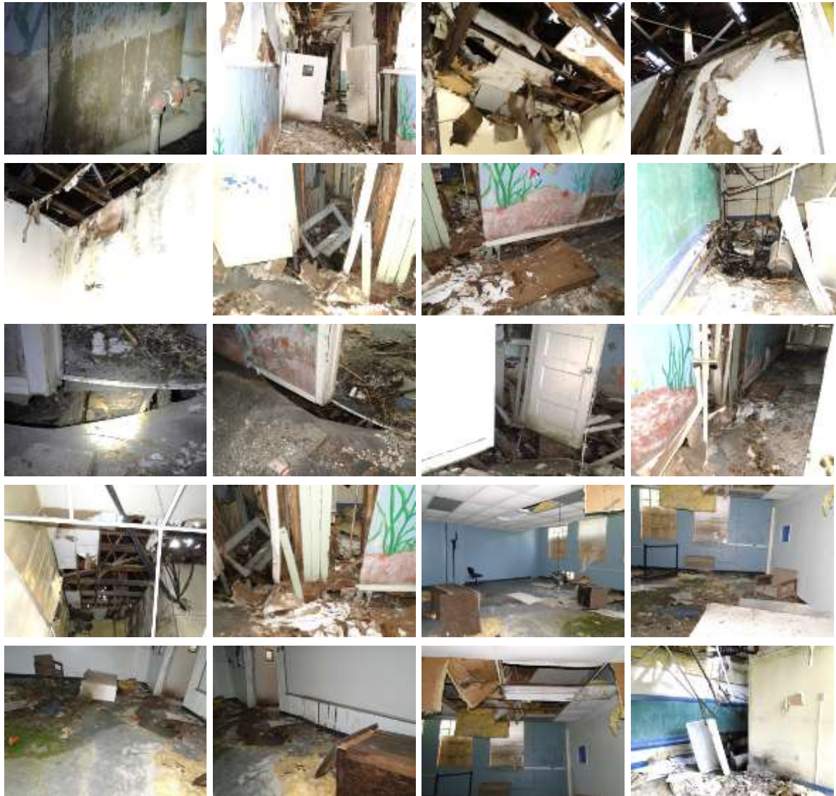
2). (Middle school addition) The addition to the middle school's floor coverings are damaged in most areas. Most of the ceiling tiles are weather damaged and a few are moisture damaged or missing. The interior floors are covered in trash in many areas.
