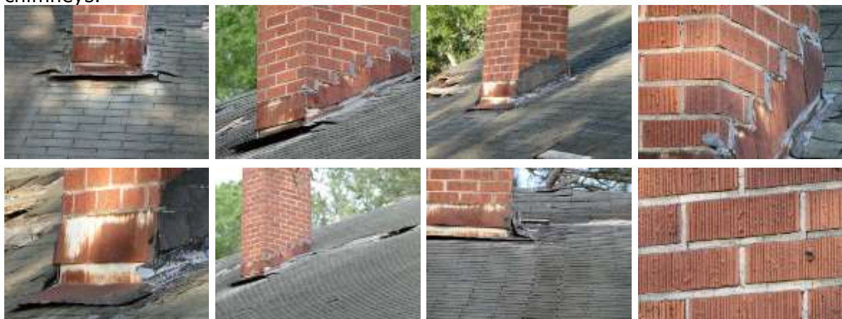
2). (Middle school) The visible flashings around the chimneys on the middle school roof are damaged and unsealed in many areas. The mortar is damaged in a few areas on most of the chimneys.
