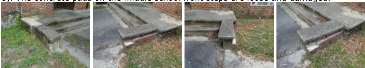
8). The concrete pads on the middle school front steps are loose and damaged.
