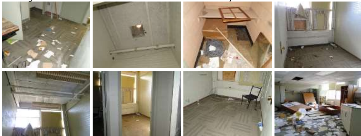
2). (Middle school addition) The addition to the middle school's floor coverings are damaged in most areas. Most of the ceiling tiles are weather damaged and a few are moisture damaged or missing. The interior floors are covered in trash in many areas.
