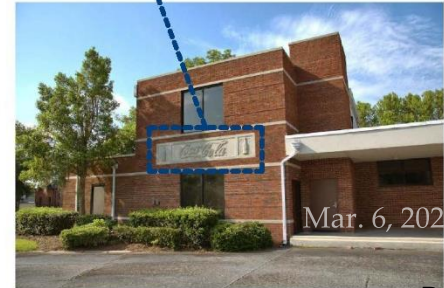
COCA-COLA BUILDING - CAST STONE MASONRY PANELS AND ACCENTS
