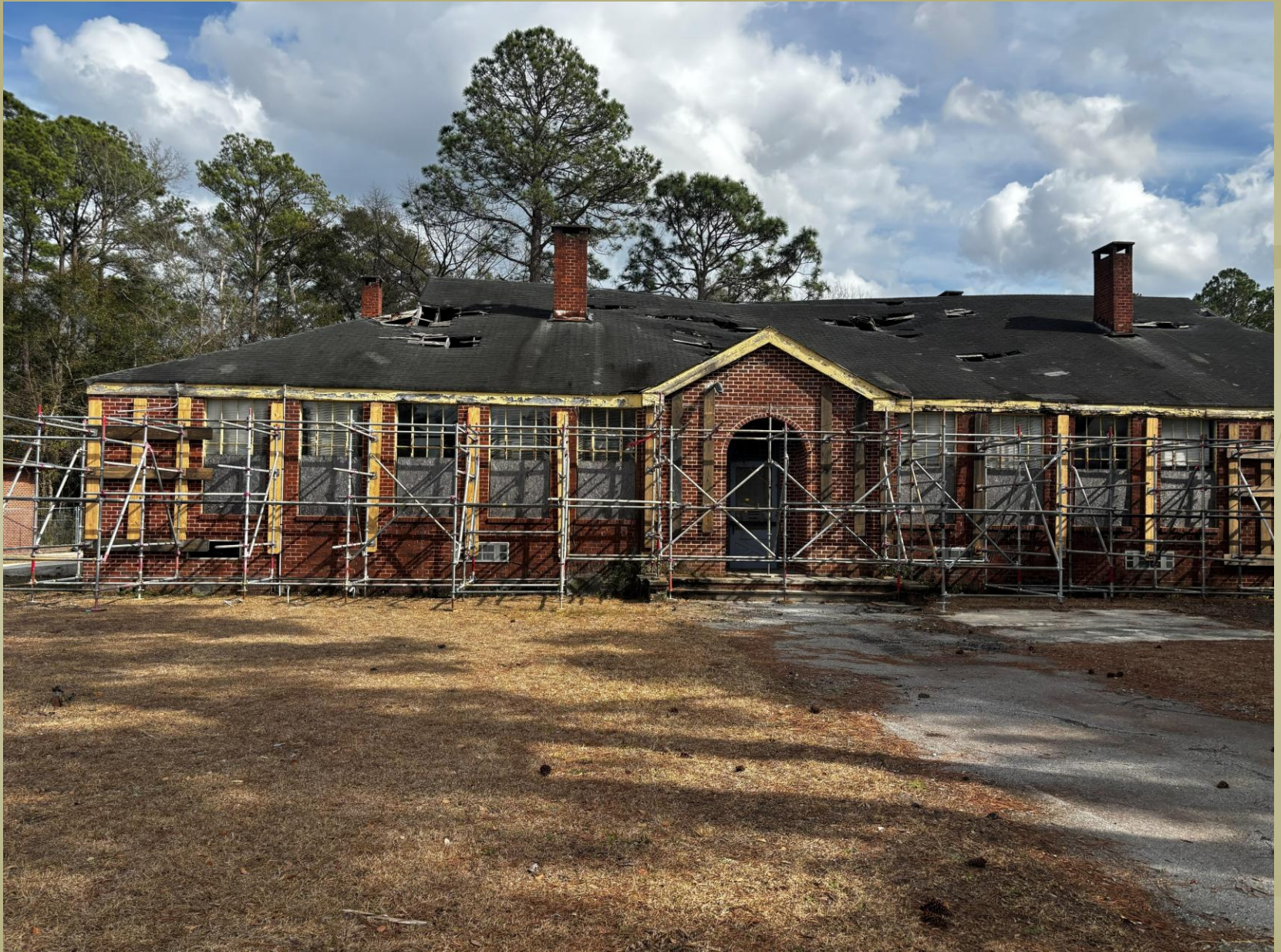
Prior to Roof Demolition
