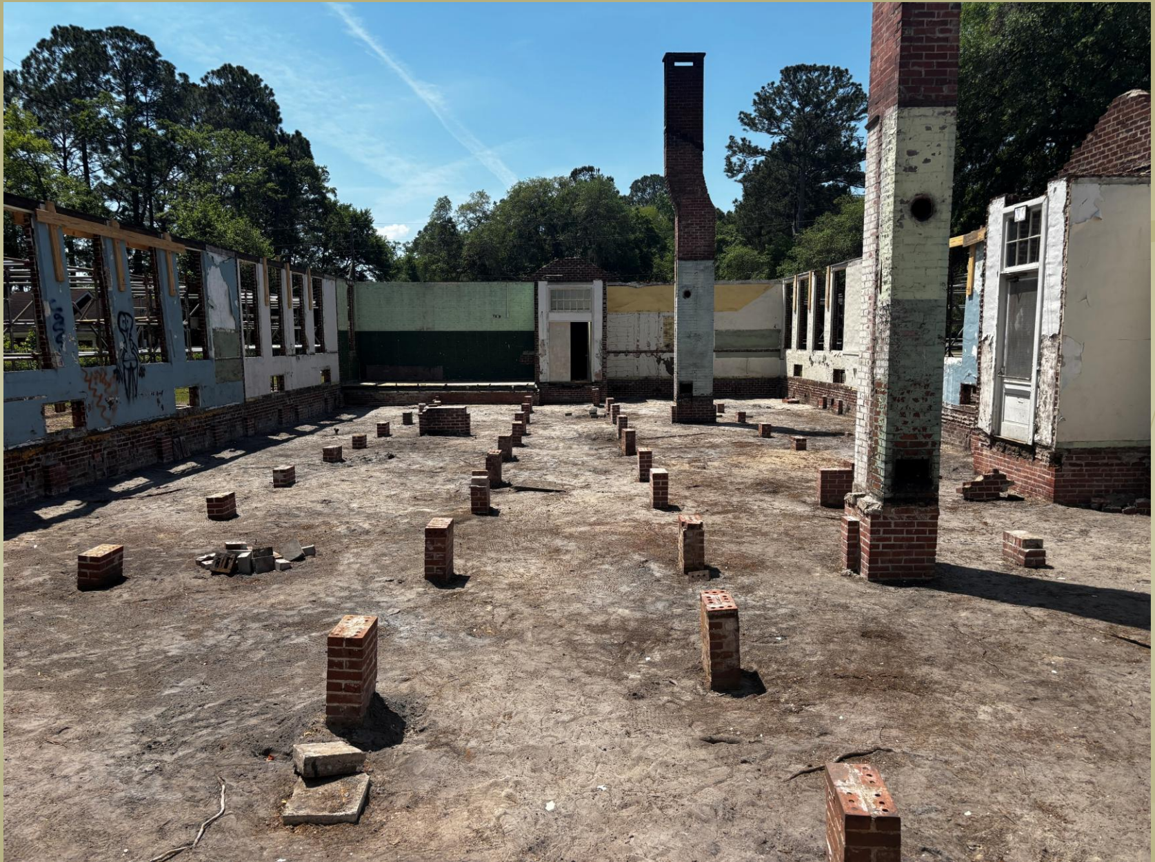
After Roof Demolition
