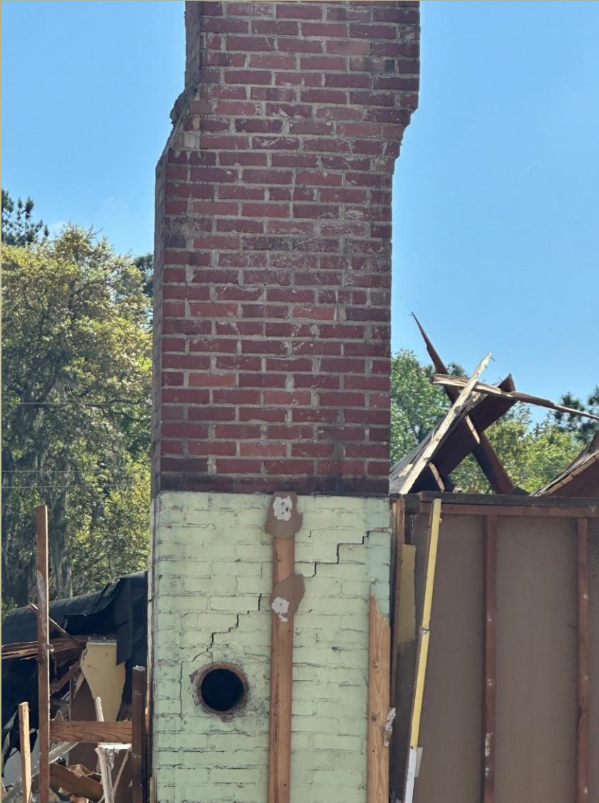
Existing Damage to Brick Stacks
