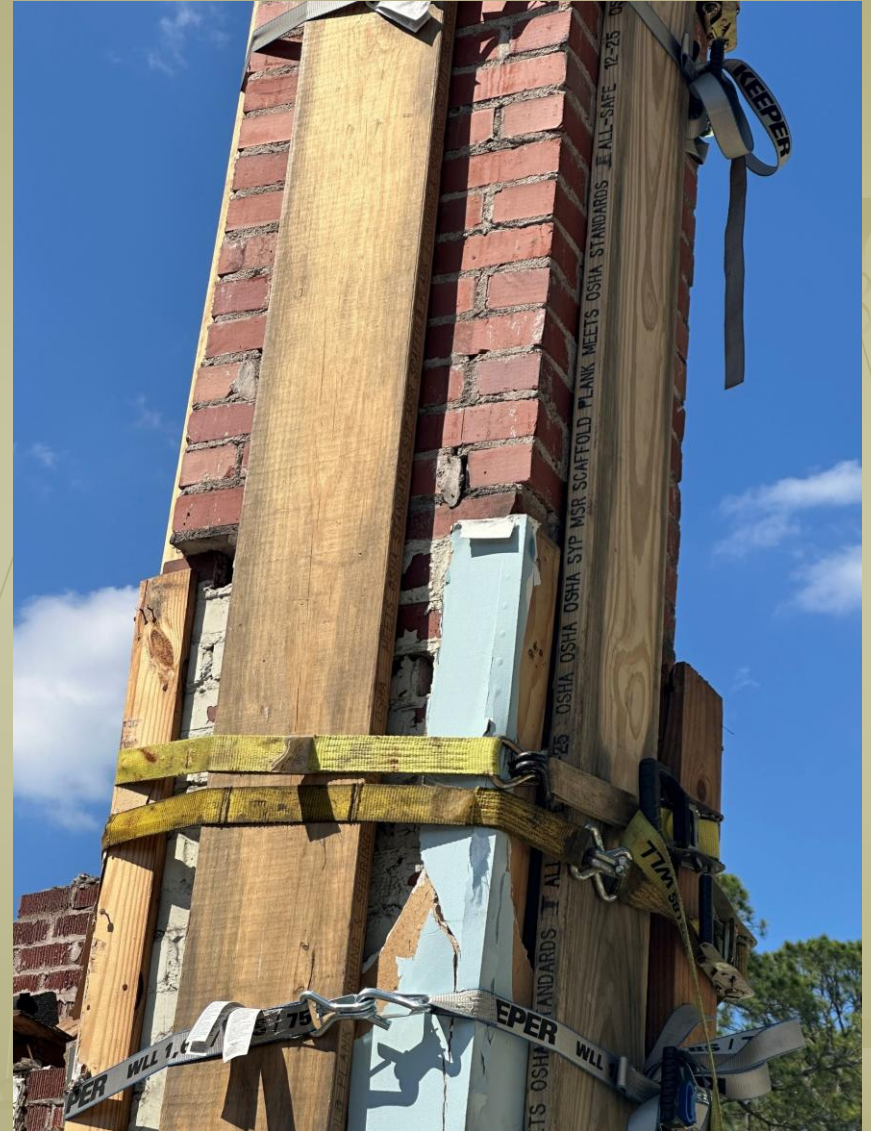
Existing Damage to Brick Stacks
