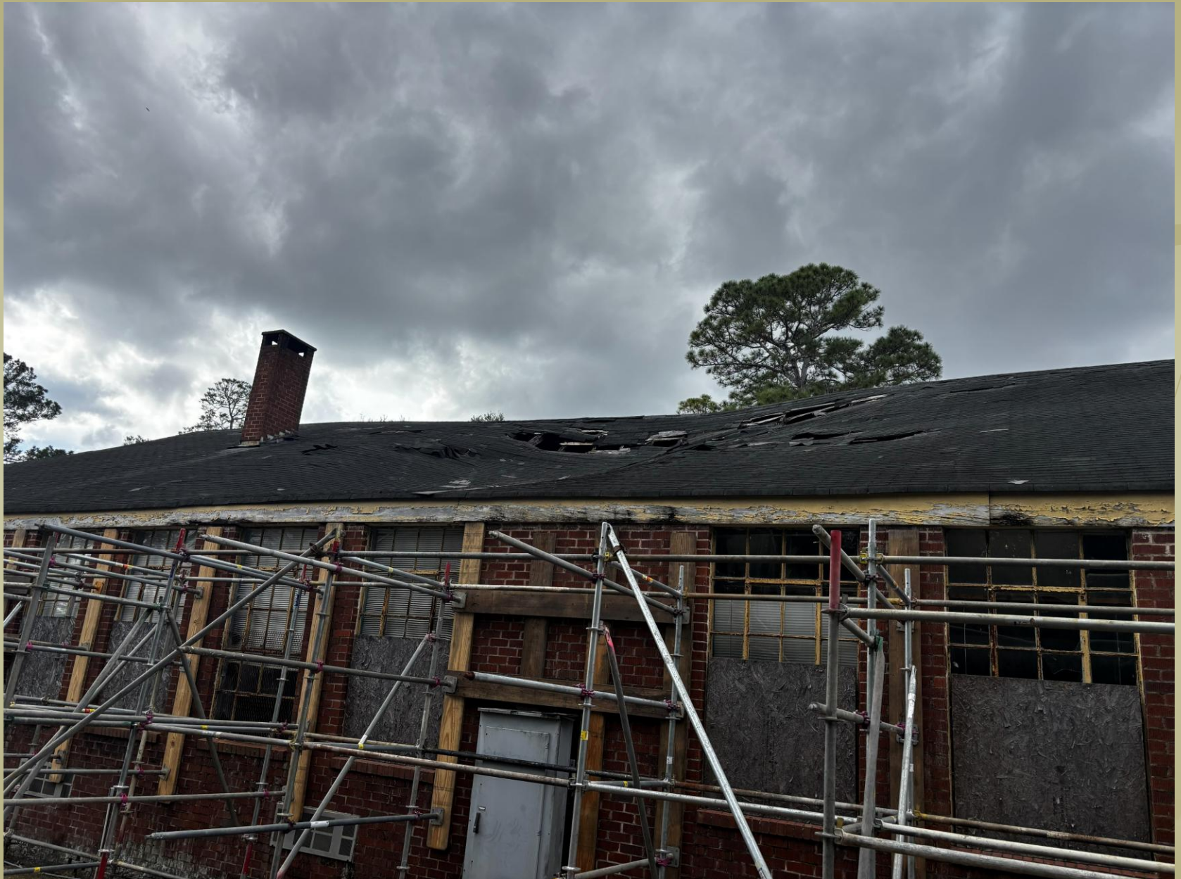
Prior to Roof Demolition
