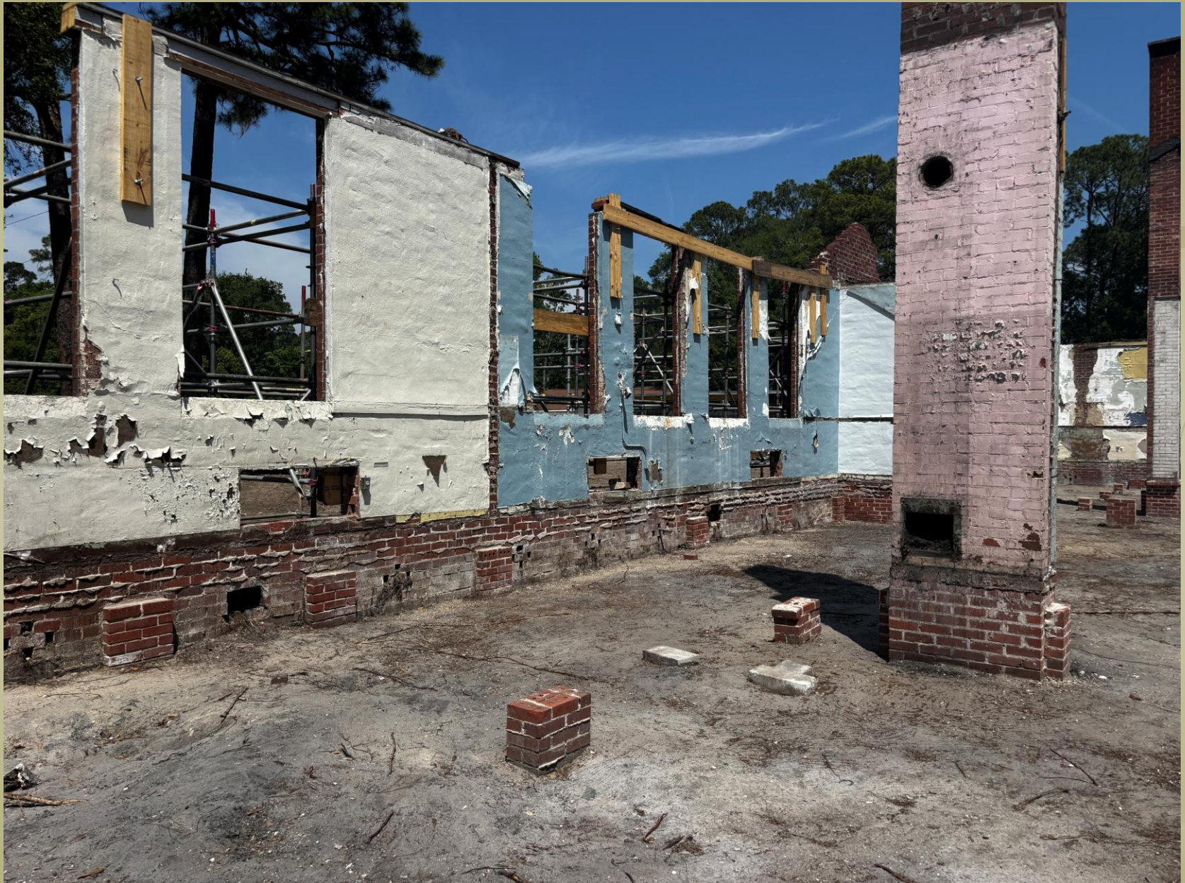
Existing Condition of Double Wythe Brick Walls
